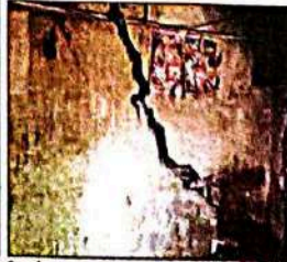
Curvilinear crack of 2-5mm wide & 2-3m long was seen on mandir floor
